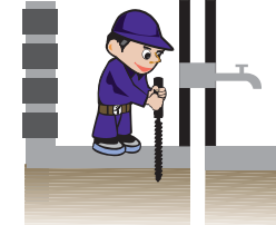
Utility Pipe Treatment
